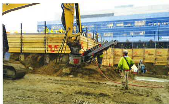
Upper: emergency stabilisation works at Hooley railway cutting, UK
