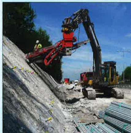
A long-reach excavator for drilling in cuttings Photo: DSI
