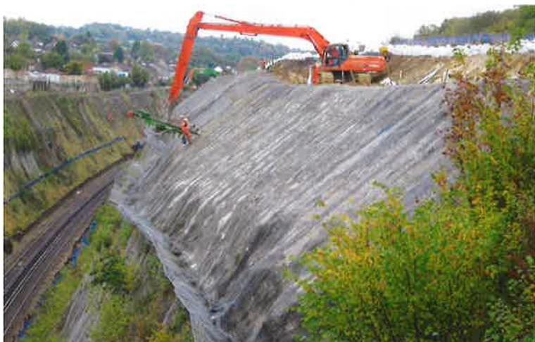
A long-reach excavator for drilling in cuttings Photo: DSI
